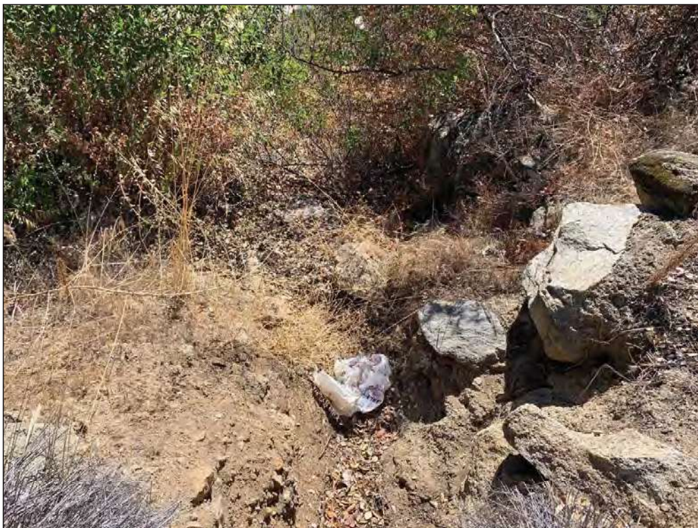
Photo Point 10: Downstream roadside culvert facing east along Mussey Grade Road
