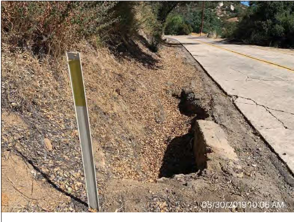
Photo Point 9: Upstream roadside culvert facing north along Mussey Grade Road.
